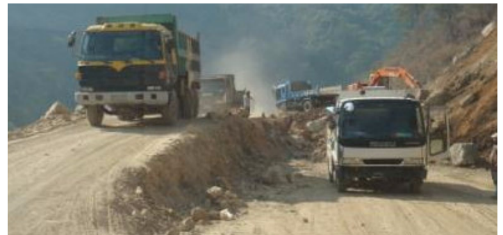
Occasional one-lane sections undergoing upgrades on the Halsema road towards Baguio.
