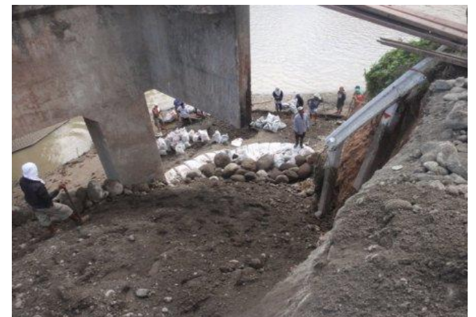
Left, middle & right views of eroded side of bridge, Dec 19. Dept of Public Works personnel working to build back retaining wall and embankment.
