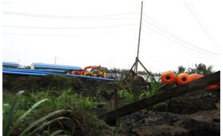
A look inside through a hole in the high sheet metal wall.
